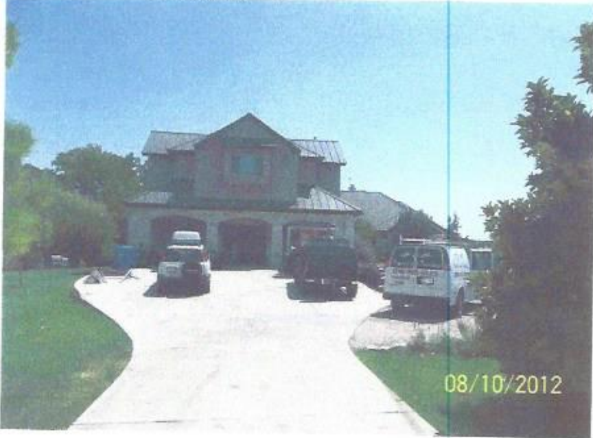
Front View – Taken on 8/10/12
